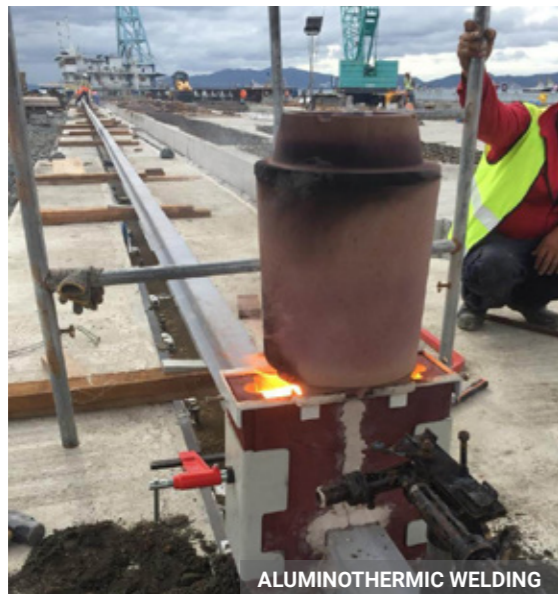
ALUMINOTHERMIC WELDING
