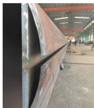
Slitting of Pipe
